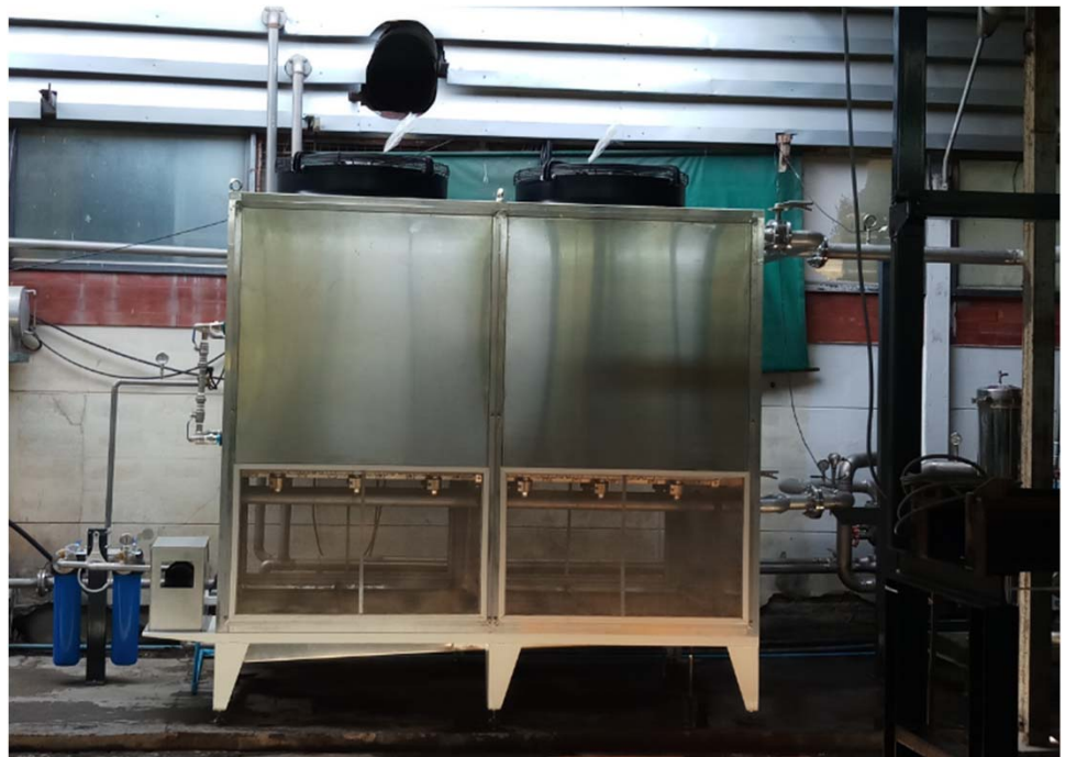
Closed circuit cooling tower (Water spray with high heat transfer cell)
